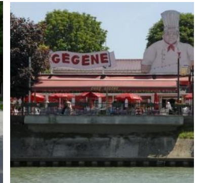
Concrete path below the street
